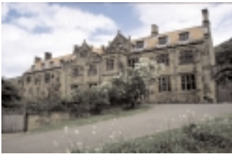
fig 5 Mount Grace Priory, showing the local vernacular detail of a pantiled roof which has an edging of stone tiles close to the eaves - Webb always made a close study of local buildings before designing a new house
