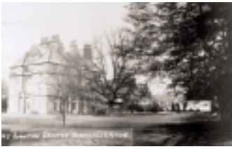
fig 4 Rounton Grange, East Rounton, North Yorkshire, one of the finest works of Philip Webb - demolished
